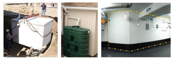
Figure 2-1. [LEFT] Pre-cast concrete tank (below ground application), [CENTRE] Plastic tank (above ground application) and [RIGHT] Cast in place concrete tank integrated within parking garage (integrated storage)<sup>6</sup>
