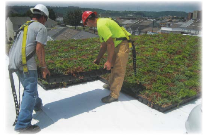
Taft Information Technology High School: A 32,000-square foot shallow vegetative roof was installed on the roof of the Taft Information Technology High School.
